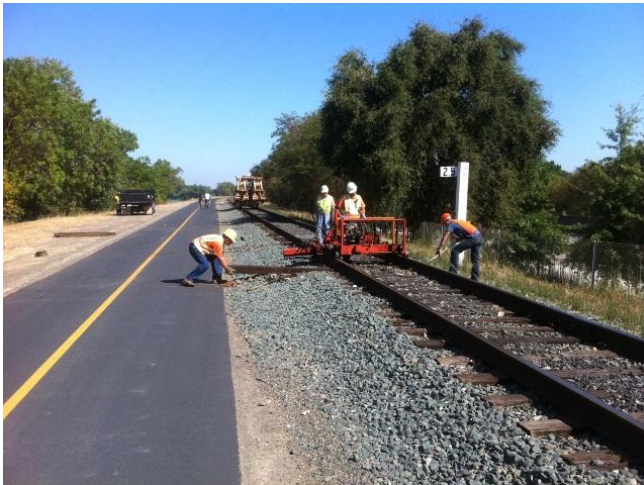
Steve moves a newish tie into position while John operates the Section Gang machine and Todd clears out some ballast. Jack is walking up to help.
