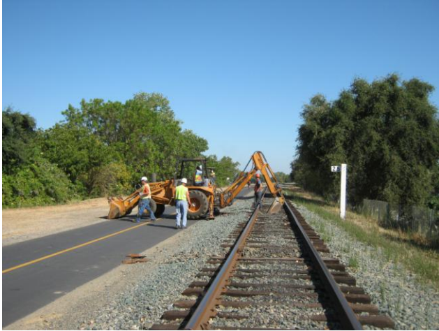
Using the backhoe to remove the old ties at M.P. 2.5. John and Jack pull out the old tie while Todd guides the backhoe.
